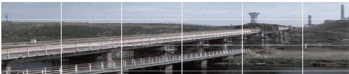
Sellafield Sea Discharge Pipebridge. Photo: CORE
